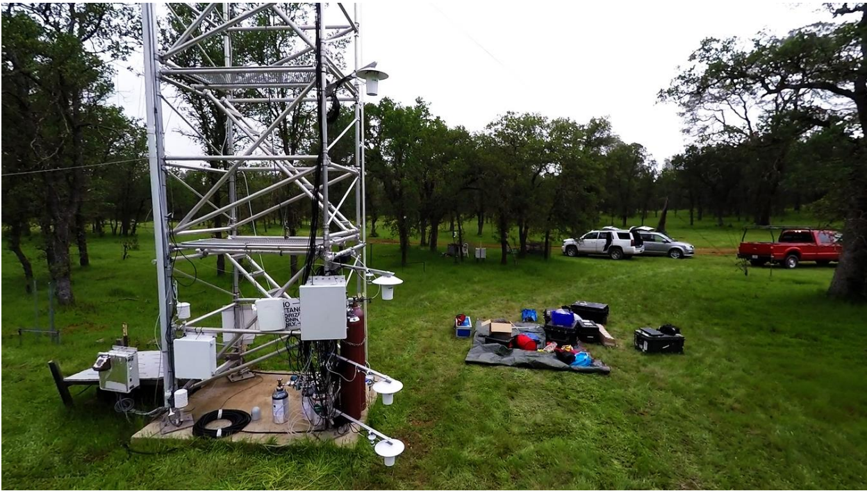
Photo 1. Main system at base of the Tonzi tower during deployment (grey box on front right leg). Inlets are located behind white aspirated temperature sensors, heights 1-4 visible. Site profile inlet 1 and 2 visible on left leg of tower.
