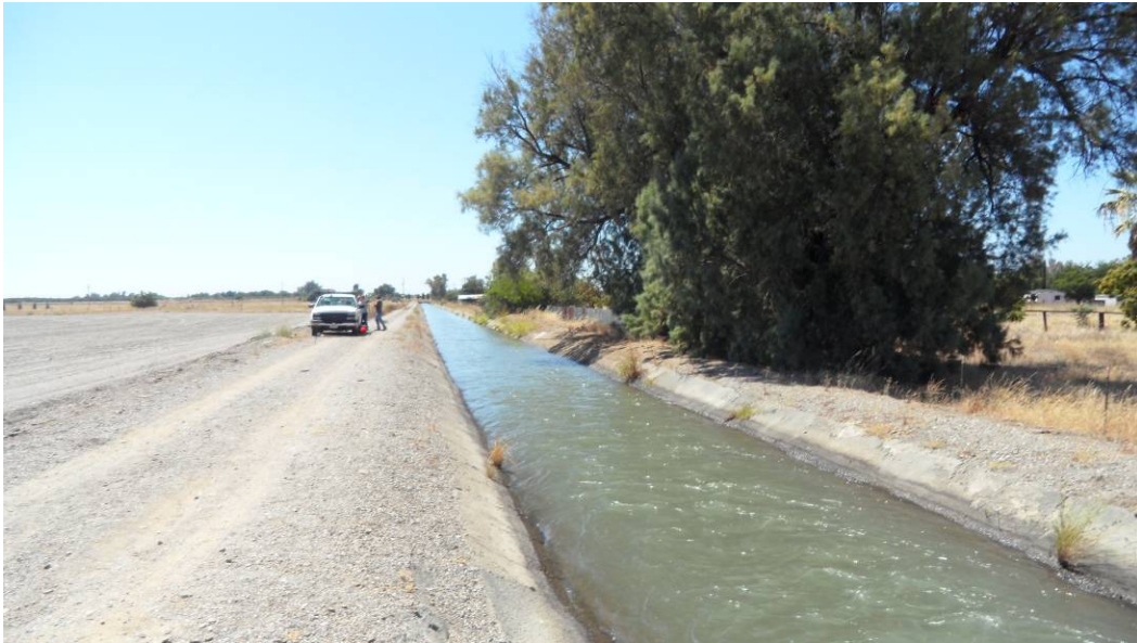
Figure 56. Example of a good installation site (long straight section of channel)
