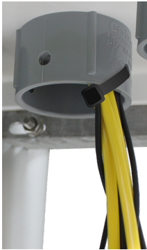
Figure 1-9. Strain relief fitting for the power distribution box. Use UV-stabilized cable ties to secure the power cables to the fitting.
